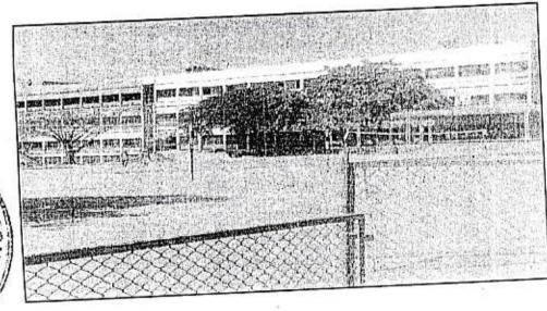
The structure in constructed as R.C.C. formed structure with brick & block masonry, flush doors, steel windows & tiled flooring.
